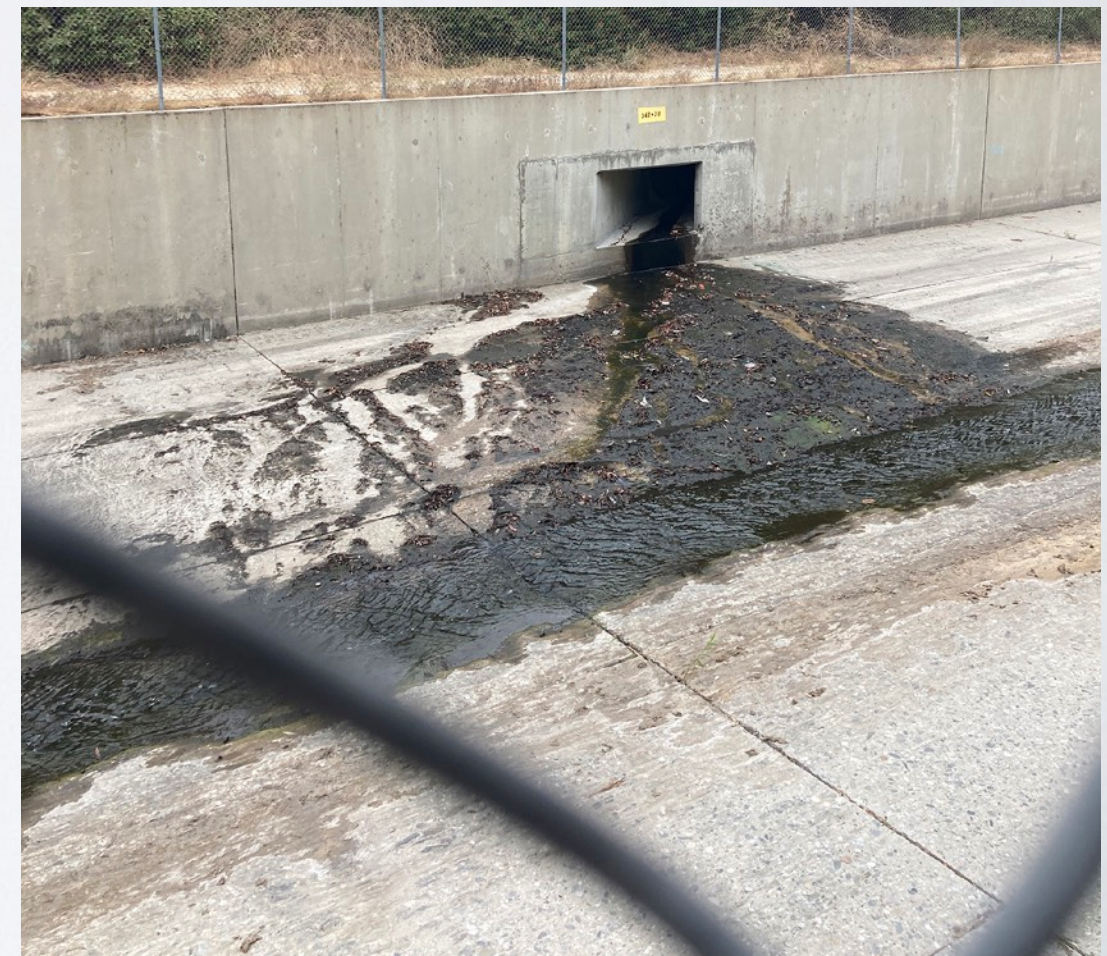
Dark muck flowing into the River
