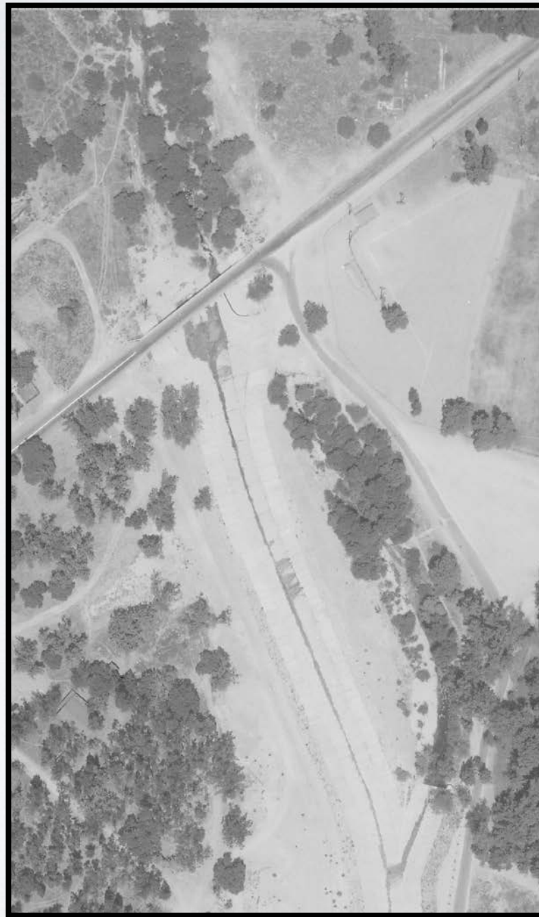
After channelization 1937 South of San Pascual ave
